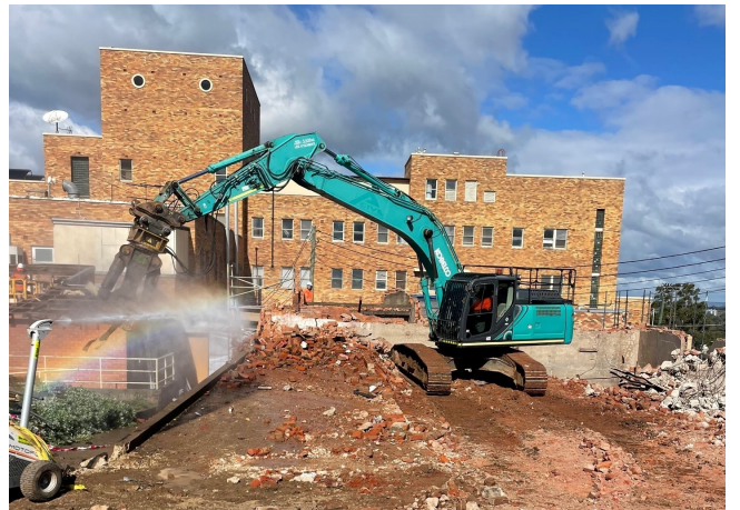
ENABLING WORKS PROGRESS
