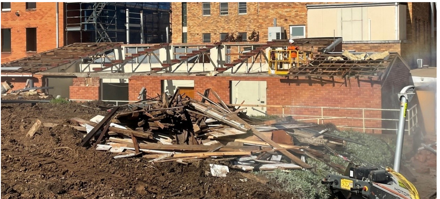
REMOVAL OF THE NURSES QUARTERS UNDERWAY
